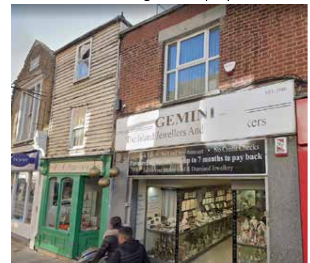
Surviving example of timber framed Weatherboarded upper floor with traditional timber shop front
