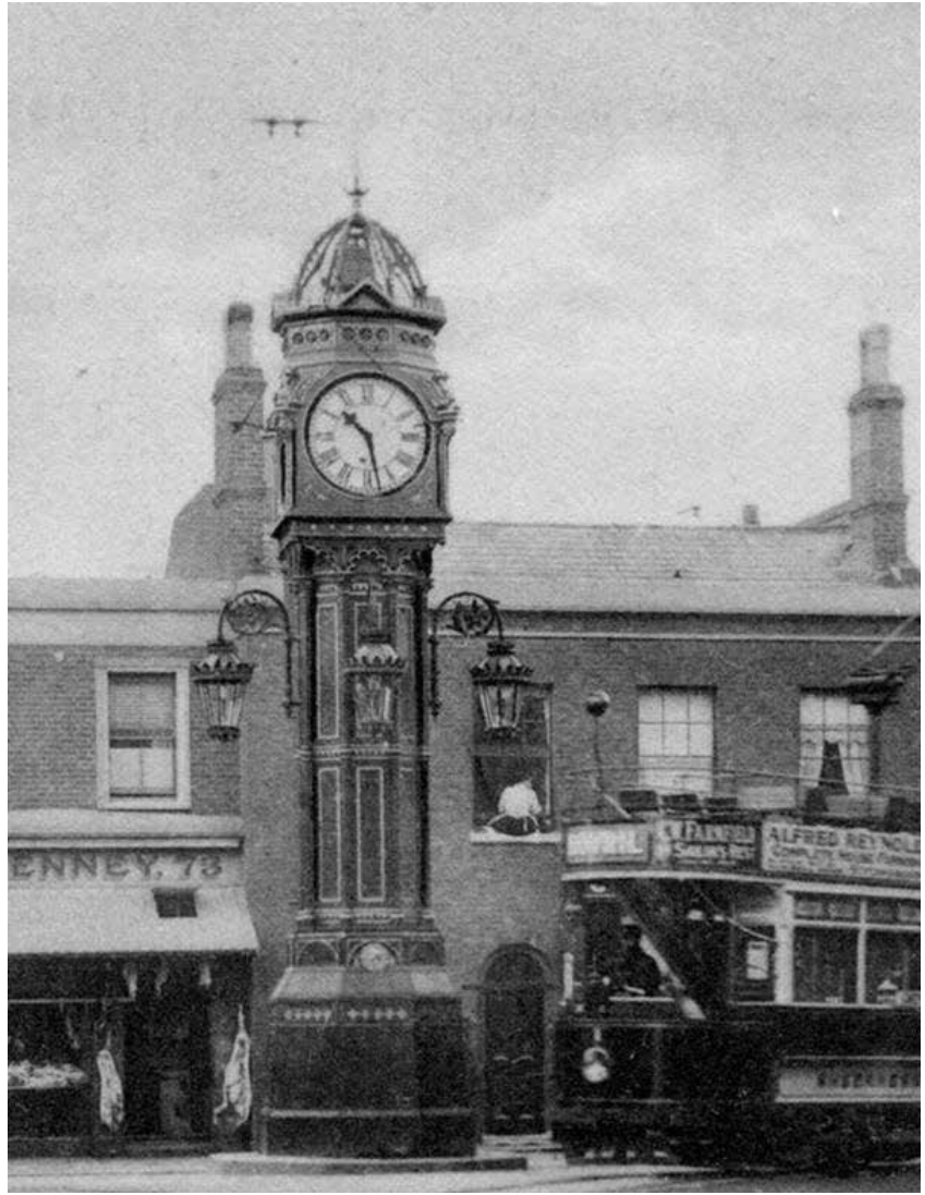
Clocktower circa 1902 with original gas lanterns- Grade II listed
