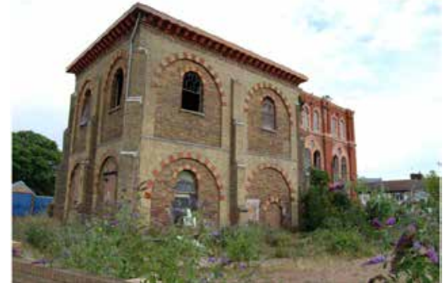
Rear view of the pumping station
